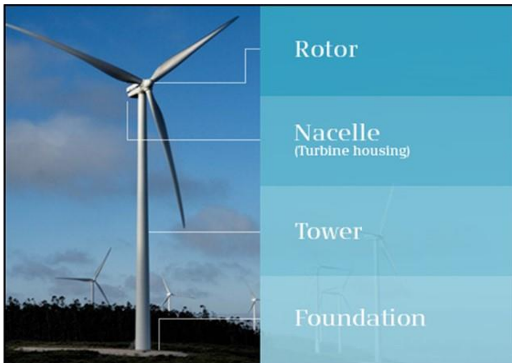
Plate 4-1 Typical wind turbine components
