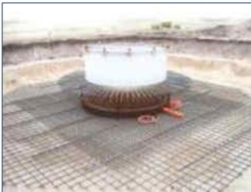
Figure 4-6 Steel Reinforcement being added
