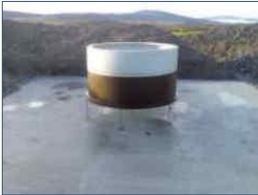
Figure 4-5 Typical Turbine Foundation Design - Levelled Turbine Tower 'Can'
